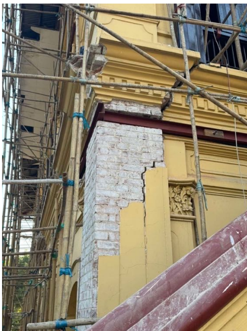
Figure 30 – Damage of corner (left) and staircase (right)
